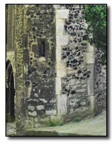
It is made even more unusual by having 'long and short' stonework which identifies it as being of Saxon construction. Sadly I have been unable to study it closely but I can see no evidence of the lower section of this little tower every having been rebuilt. This suggests to me that it was possibly the northwest corner of a bell tower and that the new C14 church was not built directly on top of the earlier one. I will reserve judgement on this until I am able to re-visit the church.
